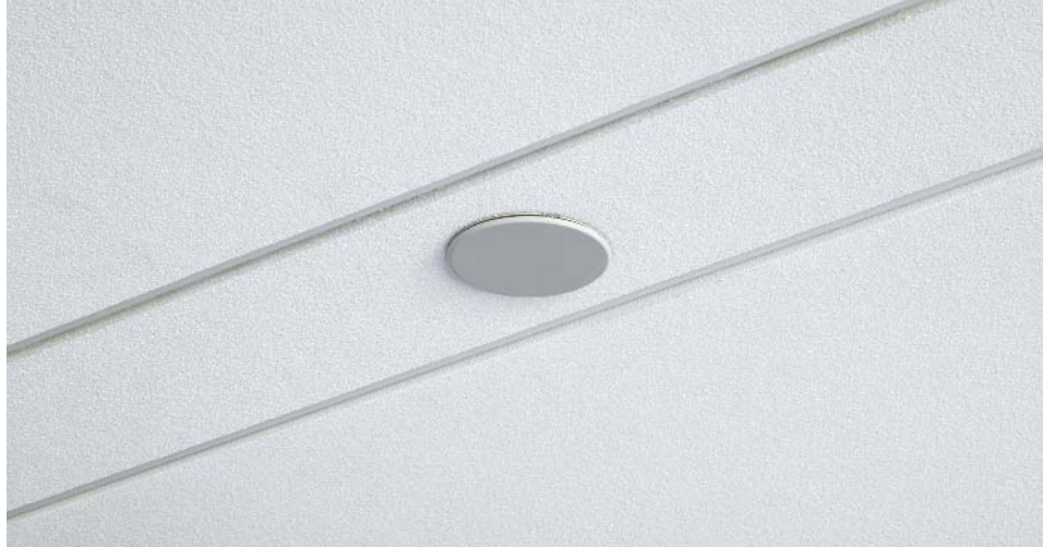
FlexHead Fire Sprinkler
