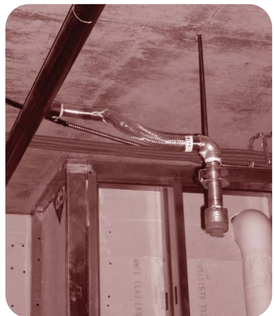
UH-2 Bracket installed with FlexHead Model 2036E
