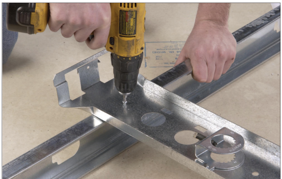
Gypsum board ceiling installation
