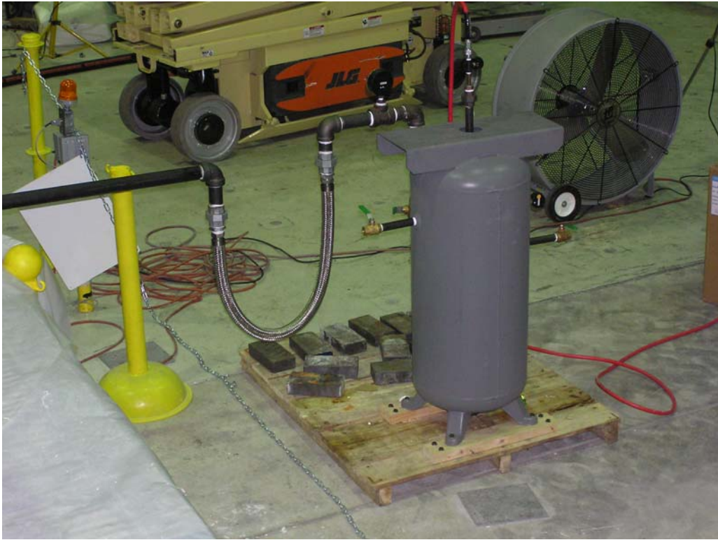
Figure 2.10 Unit used to pressurize the piping system
