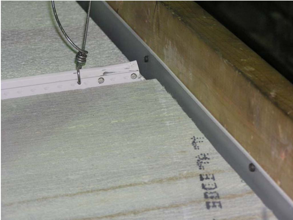
Figure 2.13 Edge connection detail in FlexHead system 1
