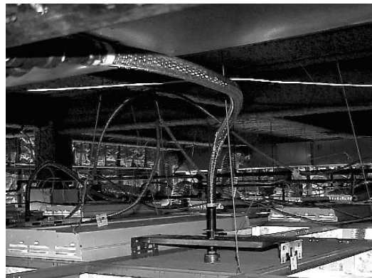
Plano, Texas retrofitted more than 4,000 center-of-tile sprinkler heads in five schools.
