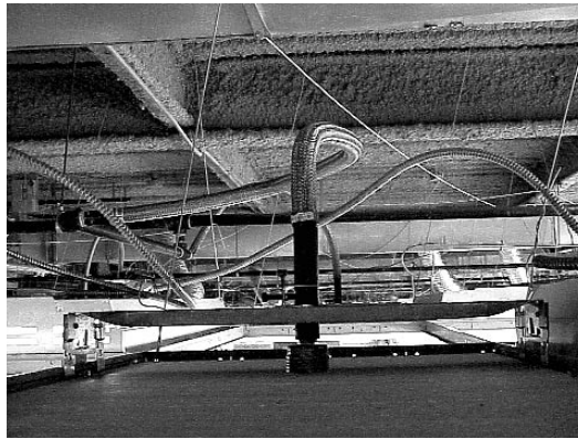
Plano, Texas retrofitted more than 4,000 center-of-tile sprinkler heads in five schools.
