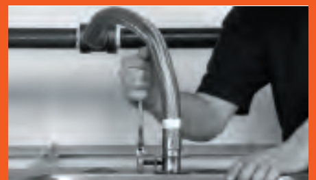
Secure FlexHead sprinkler drop to bracket.
