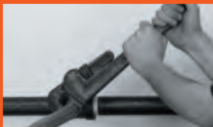
Connect FlexHead sprinkler drop to submain.
