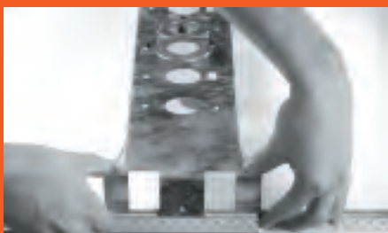
Attach bracket to t-bar ceiling grid. Connection also compatible with Sheetrock ceilings
